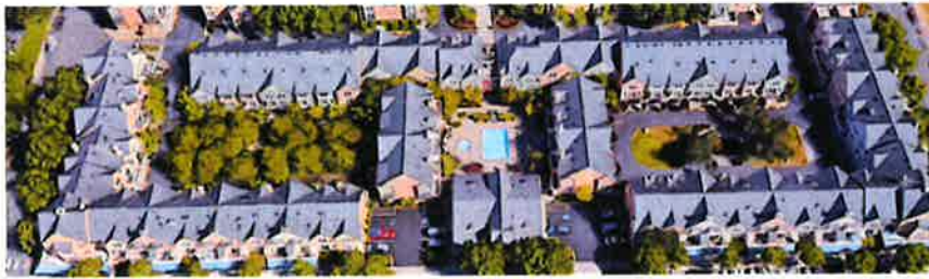
Studio apartments over ground level retail in Seattle's Roosevelt neighborhood (images courtesy of Weinstein A+U).
